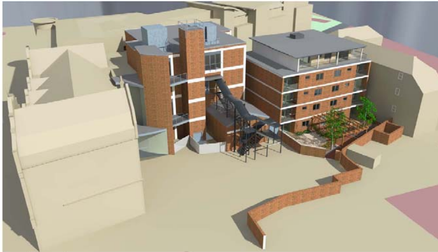
view from west
